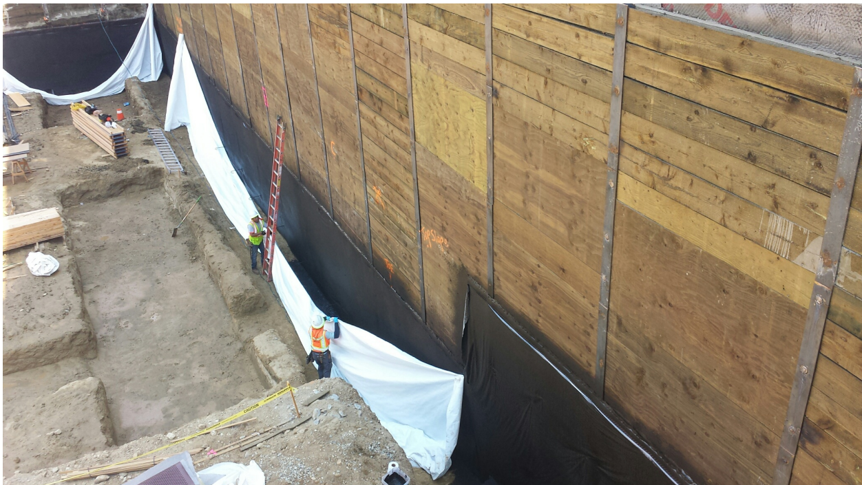
Photo: An example of wood lagging
