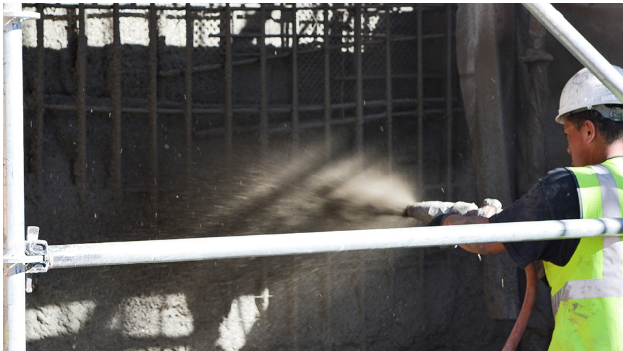
Photo: Application of shotcrete to a waterproofing system. (Photo courtesy of EPRO)
