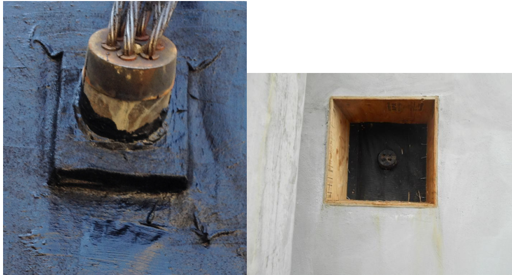
Photo Left: Tie-back sealed prior to wall placement. Photo Right: Post installation
