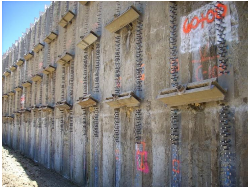
Photo: Complex shotcrete shored wall with whalers
