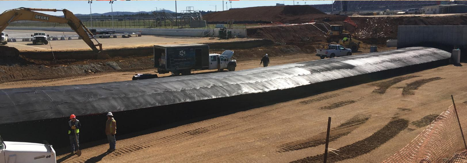
On top of tunnel: The S&H team installing 120 mil reinforced membrane as part of the E.Protect system.
