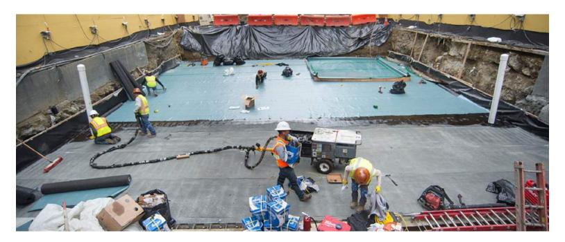
Cold fluid-applied polymer rubber gel composite membrane system Self-healing, non-curing, flexible, versatile
