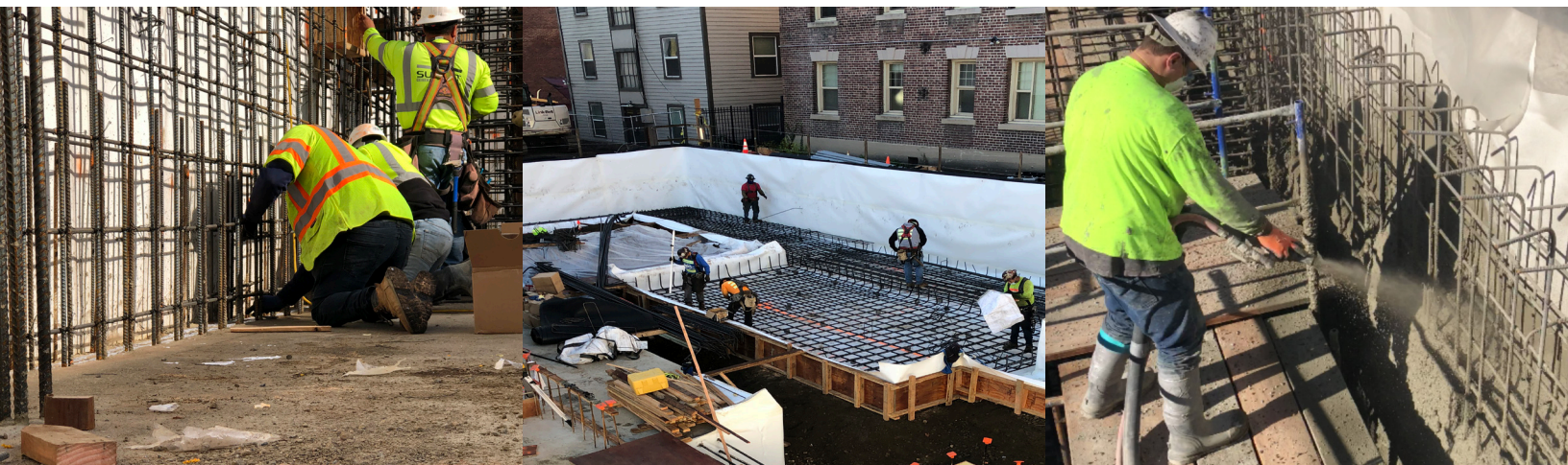
Installation of rebar against vertical blindside application of the PreTak membrane.
