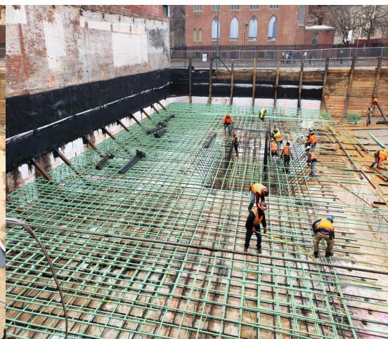
Rebar installation after system installation is complete.
