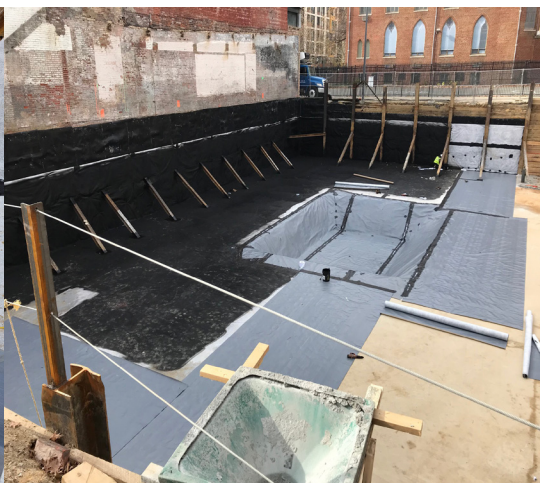
Installation of Geo-Seal® BASE and Geo-Seal® CORE on underslab and below grade walls.
