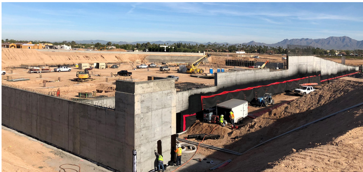
Application of E.Protect at first lift.
