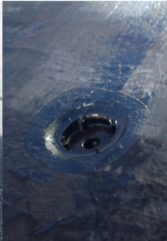
Detailing deck drain
