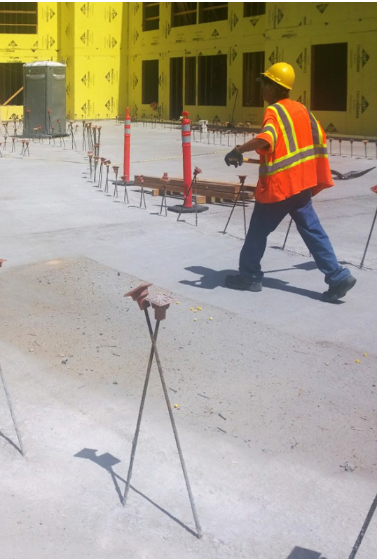
Deck prior to application of E.Protect Deck application
