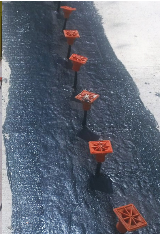
Application of reinforcement detail around penetrations
