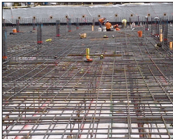
Structural Slab with Blind-Side Walls
