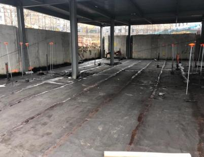
Structural waterproofing was needed for 40,000 square feet of underslab waterproofing and 10,000 square feet of post-applied wall to prevent water and vapor intrusion. Multiple grade beams, elevator pit and sump were completely enclosed in the E.Protect underslab waterproofing system. The stepped perimeter footings were also wrapped with the system up the side of the footing form where it then transitioned to E.Protect+ Wall for the post-applied, positive side vertical waterproofing application.
