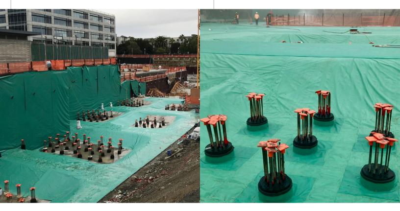
An additional challenge arose because the foundation was secured in place by auger cast piles.
