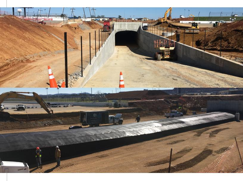
On top of tunnel: The S&H team installing 120 mil reinforced membrane as part of the E.Protect system.
