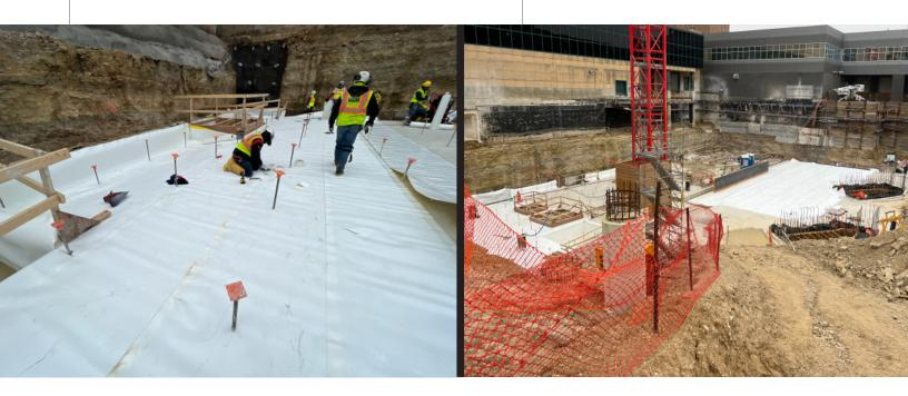
PreTak is a pre-applied high-density polyethylene (HDPE) sheet waterproofing membrane combined with a pressure sensitive adhesive that fully adheres to cast in place concrete and shotcrete to prevent lateral water migration in both blindside shoring and underslab applications. Installation is productive and reliable with up to 8 ft wide rolls to minimize seams.
