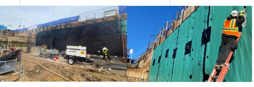
running directly across the bottom of the elevator pit, flooding the area where the under slab and pile caps had to be detailed water and vapor tight. Through a collaboration between EPRO's technical team, Osprey's experienced application team, and the GC, HITT Construction, we were able to determine how to safely and efficiently redirect the stream's flow to allow for a warrantable waterproofing installation."
