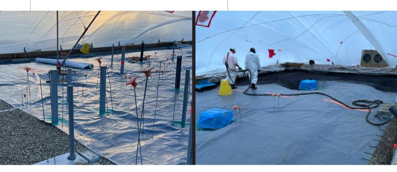
Collin Watson, also of EHI Projects, added, "When the original Zoo project was presented to us, we accepted its 9,200 square foot liner installation combined with a complex perimeter seal, along with an additional 400+ liner mechanical penetrations as another day at the office. We could easily see why the environmental design engineers, WSP, chose EPRO products and particularly Geo-Seal 100 as the product of choice."
