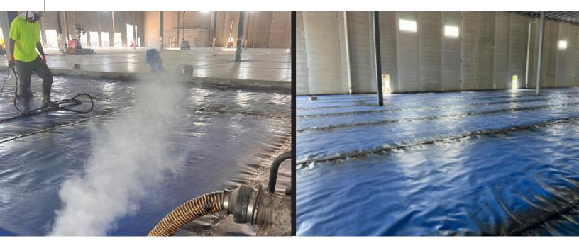
"We installed the entire passive vapor mitigation system which included, but was not limited to, Vapor Vent piping, passive remote monitoring probes, and EPRO's Geo-Seal EV40s," says William Stetson, Project Manager, Edgeboro International, the EPRO installer. "We are very familiar with EV40s and use it frequently. It is easy and quick to install over large areas, such as this facility."
